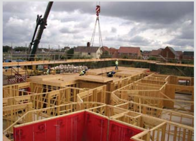
Development under construction
